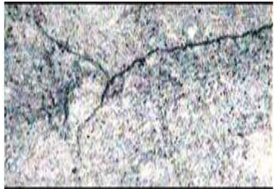
Figure 4: Blood Transfusion Centre, Serology Laboratory, coating of Portland cement
